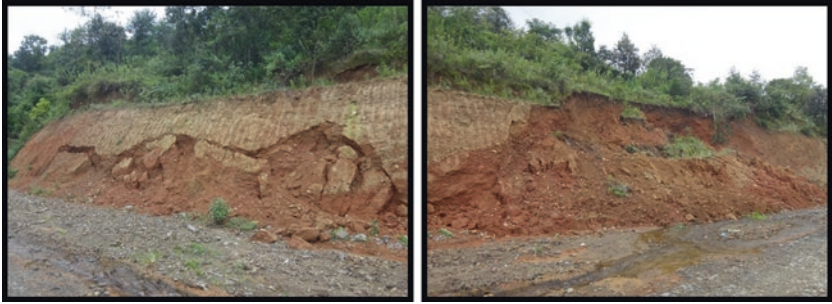
Fig. 12.5 Residual soil occurring along the slope of road section
