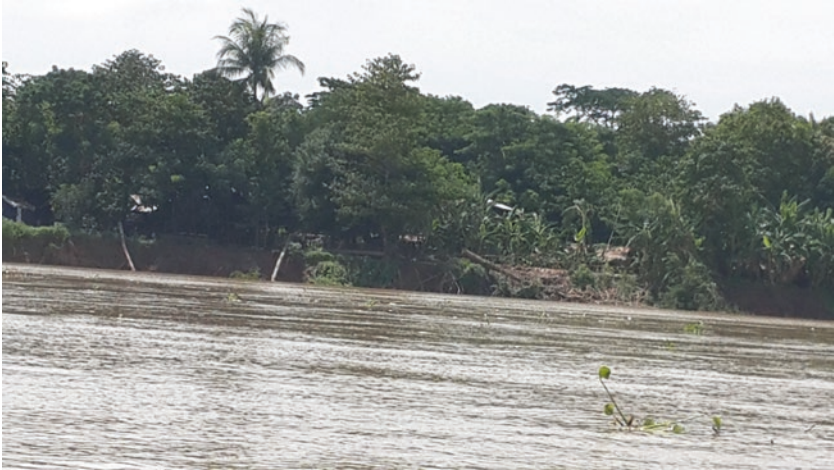
Fig. 6.1 Bank erosion in some parts of Nyaungdon Township. (Source: Photo by Wint Wint Htun 2016)
