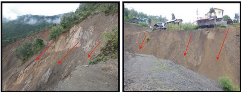
Fig. 12.7 Photographs of slope failure due to steep slopes
